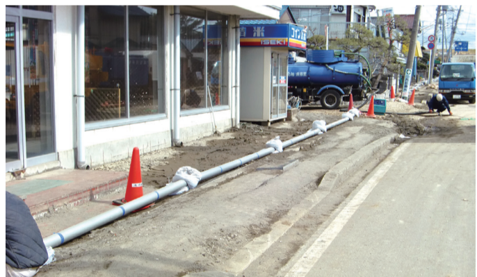
▶ 仮設配管布設状況
